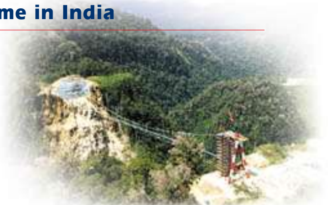
Hegigio George Suspension Bridge at Papua, New Guinea. [World's longest pipeline suspension bridge supported by Usha Martin galvanized PE coated (bonded) LRPC strands]
